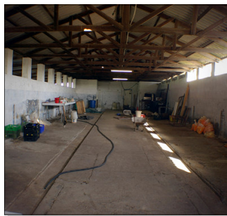
Church meeting place before renovations.
