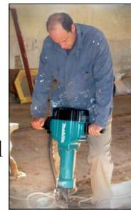
Gerhard on a jackhammer.
